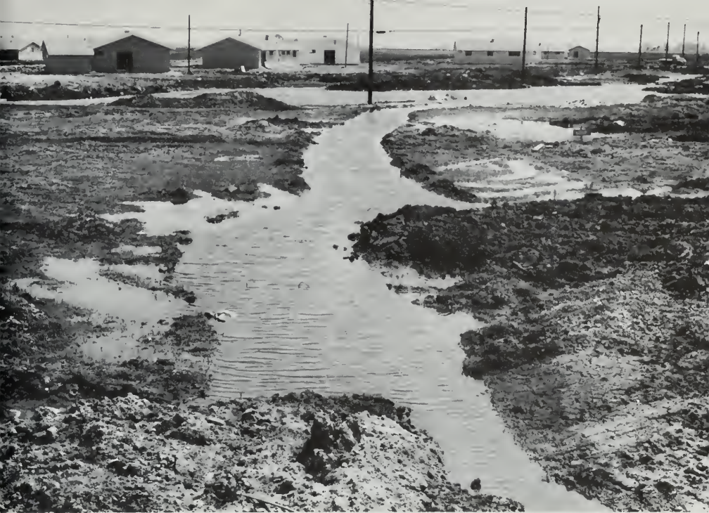
Poor drainage is manifest in this subdivision in Cook County in Illinois.
